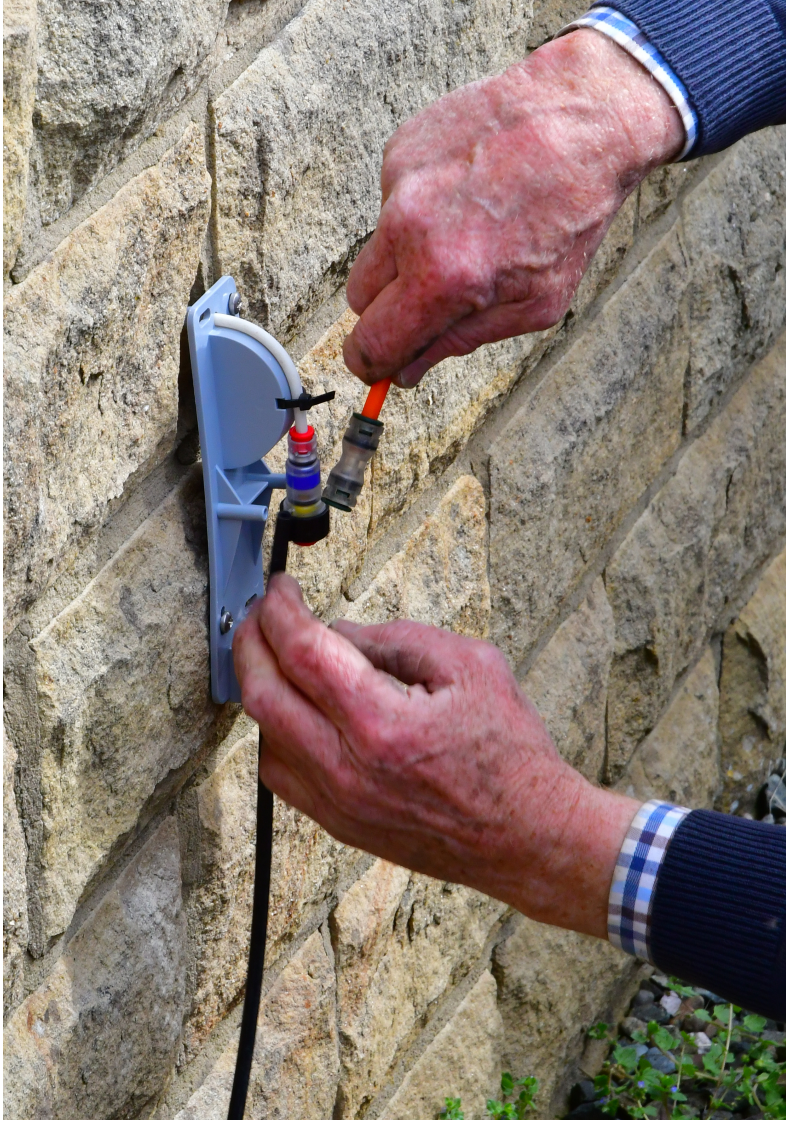
Fibres being installed in a wall box
